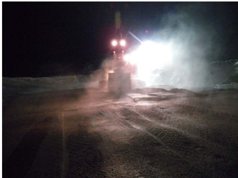
Photo 13: CAT 325 excavator placing FCM.
