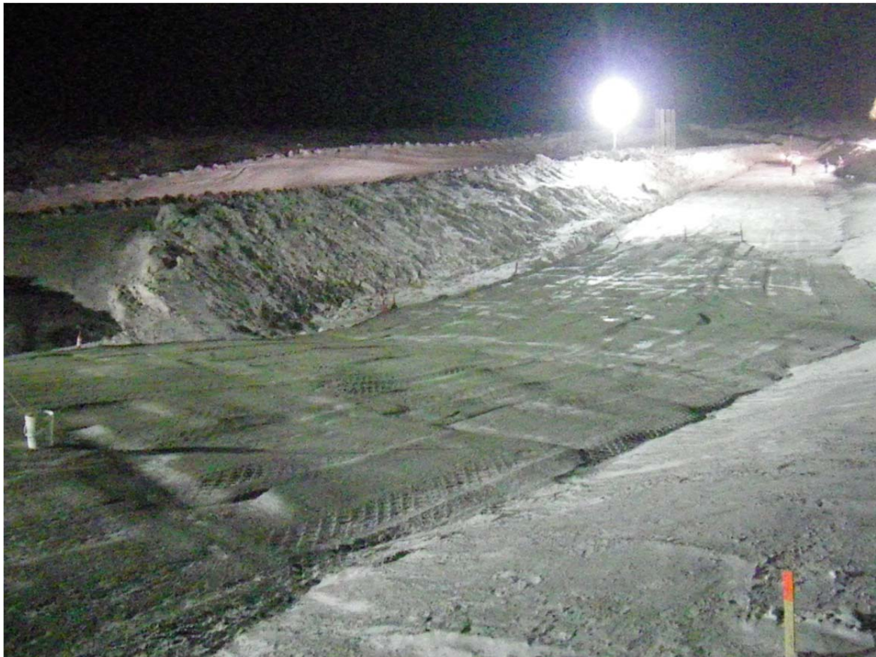
Photo 11: Placed FCM looking NE along key trench from ~station 0+60. Placed material ends where the photo transitions from grey to white.
