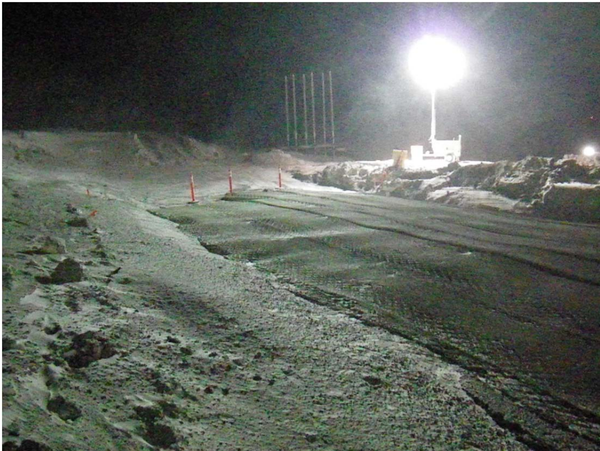
Photo 10: Placed FCM looking west along key trench from approximately station 0+60. Material placement ended at the delineators ~sta. 0+40.
