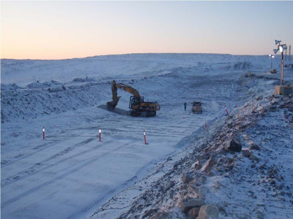
Photo 1: ~ SSW view of the 325 excavator (with finishing bucket) cleaning the upper side slopes of 5/8" material around 1+10.
