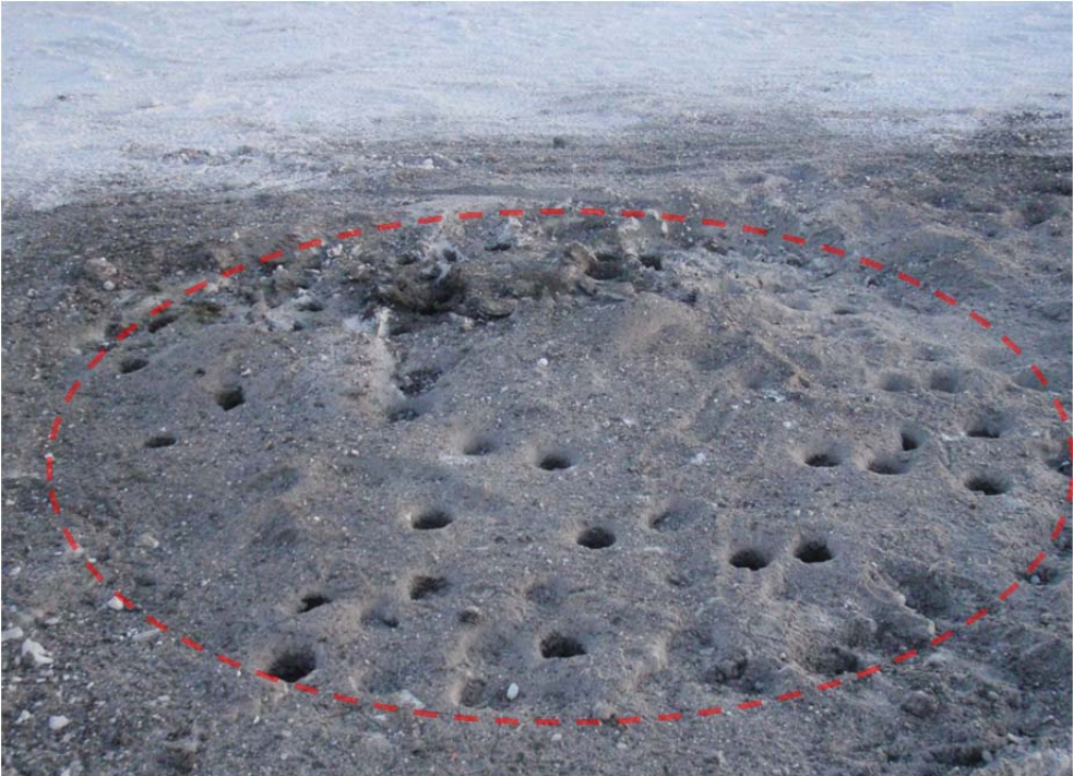
Photo 2: Close-up view of the Sump #2 location after drilling was completed. Note that some of the drilled holes are not visible due to the cutting in the area. The Sump location has a 'honeycomb' appearance
