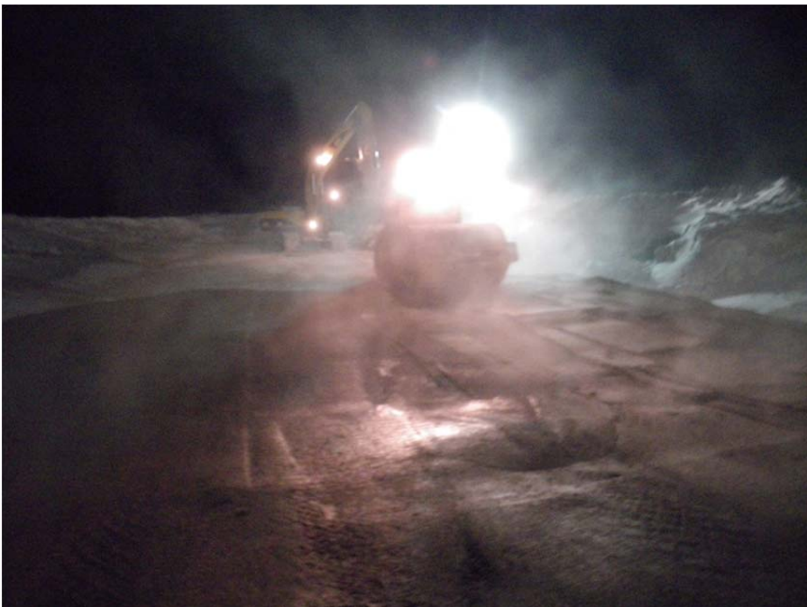
Photo 14: Packer compacting the placed FCM. Looking SW along key trench.
